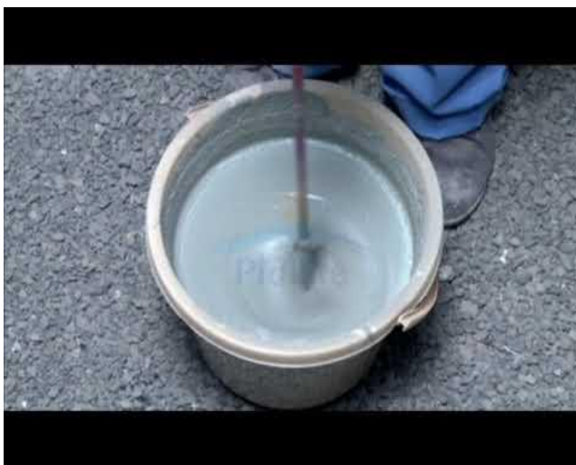
Fig2; Mixing of DR. FIXIT PIDIFIN 2K 112.
